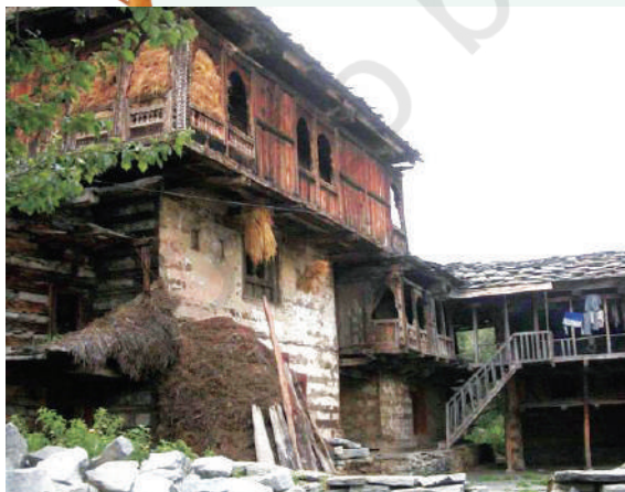
Fig. 1.6. Kath-kuni House, Himachal Pradesh
